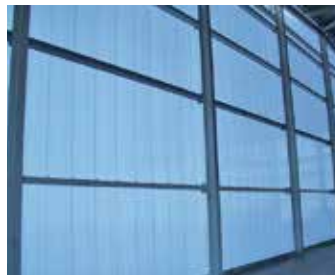
7 Haestens Office Building in Sweden LEXAN THERMOCLICK sheet system
